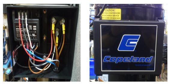
Figure 15: Correct electrical installation with cable glands for IP54 T-box (models TW\*)
