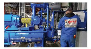
Because of its higher capacity, one Vilter  $CO_2$  single screw compressor replaced the existing two reciprocating  $CO_2$ compressors. In fact, the cooling capacity of a  $CO_2$  single screw compressor is 830 kW at -40 °C (-40 °F) evaporation and -7 °C (19 °F) condensation temperatures—nearly doubling the capacity of its predecessors. Ideal for subcritical  $CO_2$  applications, the Vilter  $CO_2$  single screw compressor now serves as a reliable anchor for the low side of the system.
