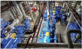
The system still uses the original four Vilter ammonia compressors on its high side. For added reliability and continuity during scheduled maintenance, the system was designed to repurpose the previous reciprocating  $CO_2$  compressors in a backup role.
