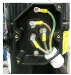
Figure 26: IP54 T-Box and correct electrical installation with cable gland
