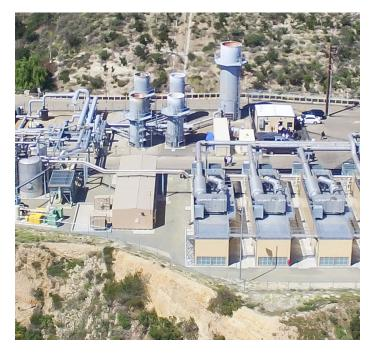
Dehydration equipment is necessary to ensure that the moisture does not cause any freezing problems during pressure changes and prevents any damage to components due to carbonic acid forming.
